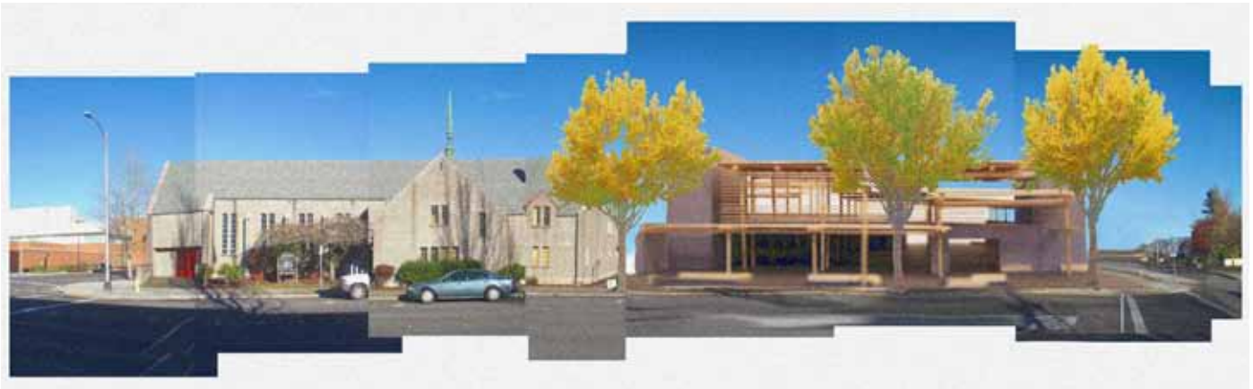
Figure 45: Looking north across A Street (Collin Janke).
