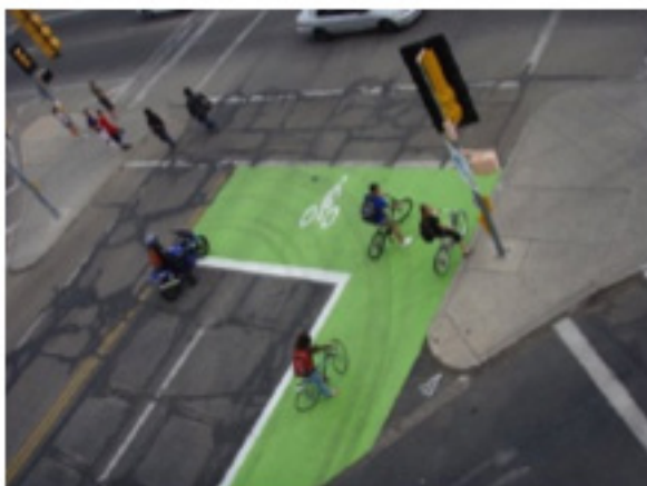
Figure 12: Bike boxes allow full visibility of the bicycles in front of the car traffic, priority signals allow cyclists to proceed before vehicular traffic.
