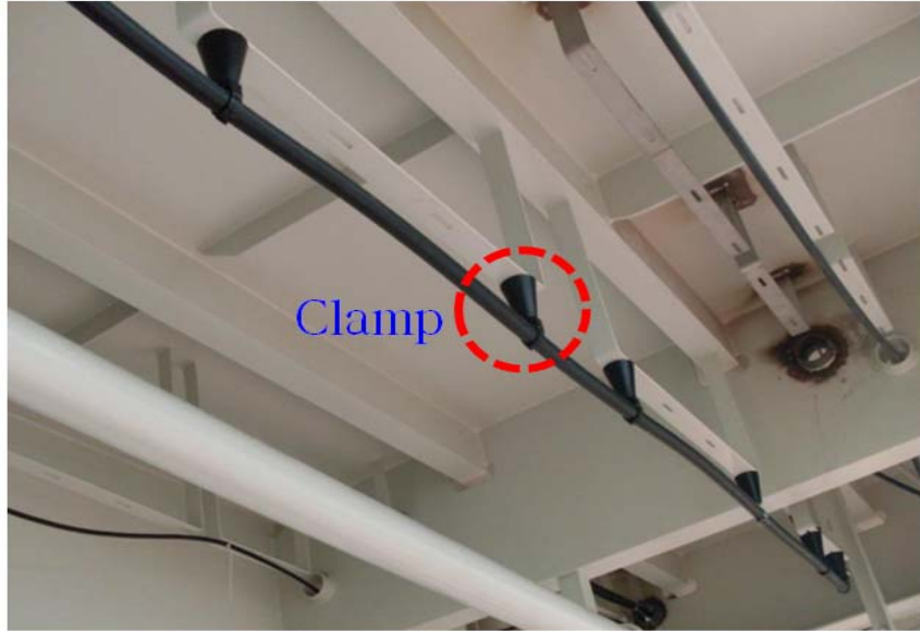
Fig. 5.11 Installation of Leaky antenna
