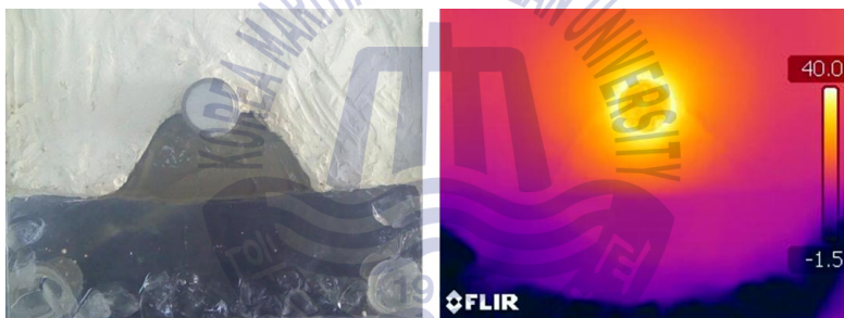
(a) Picture & Thermal image of 'E41'
