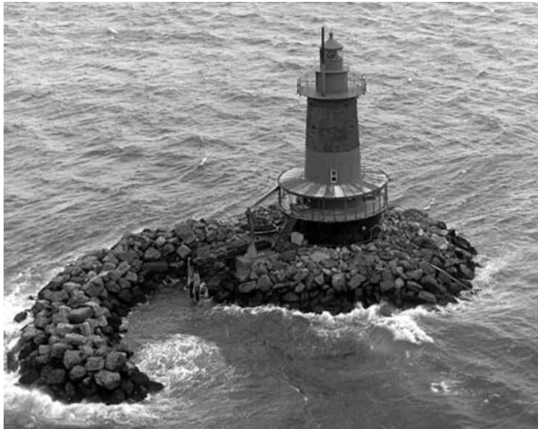
Fig. 71 West Bank Leading Light (Front) 1901~Current
