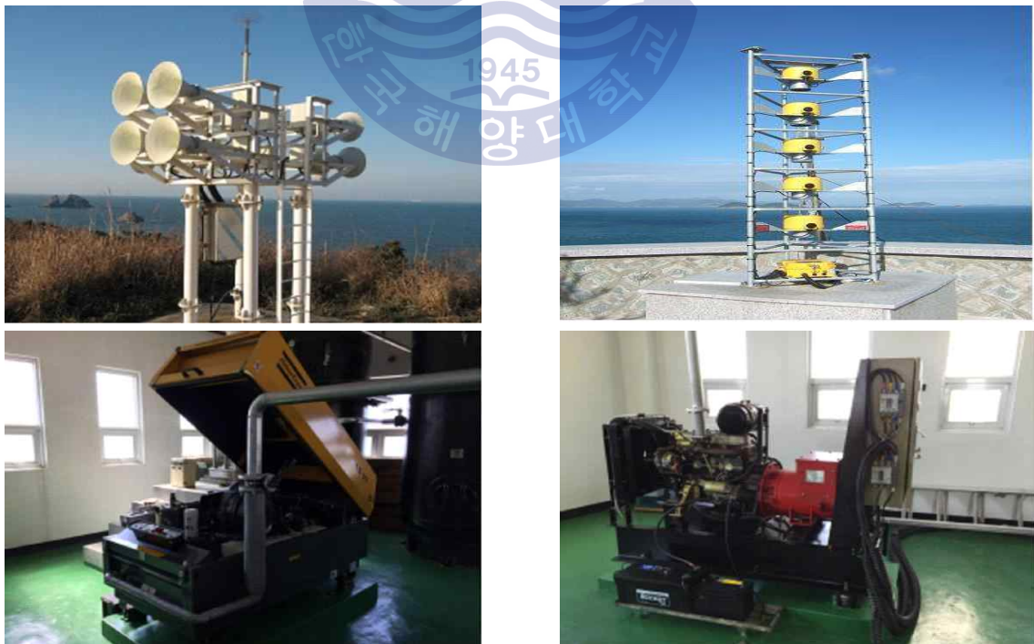
Fig. 26 Air Siren, Electric Horn and Generator
