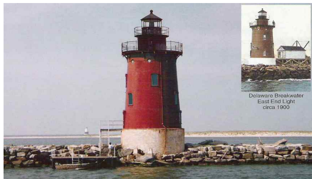
Fig. 73 Delaware Breakwater East End Leading Light(Front) 1885 ~ Current
