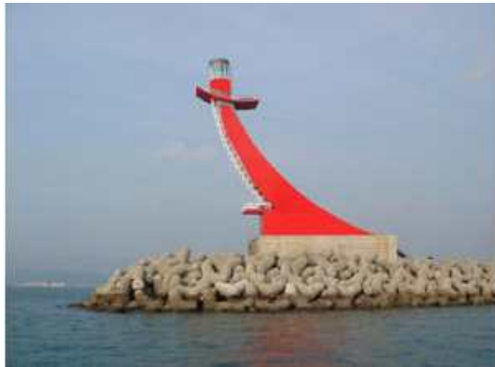
Fig. 7 Unmanned Lighthouse in Busan New Port Breakwater
