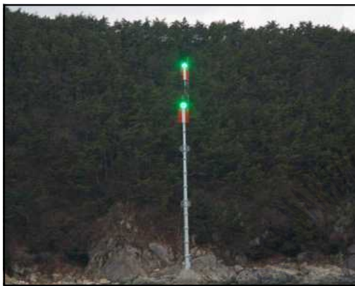
Fig. 48 View of Busan New Port Songdo Leading Lights
