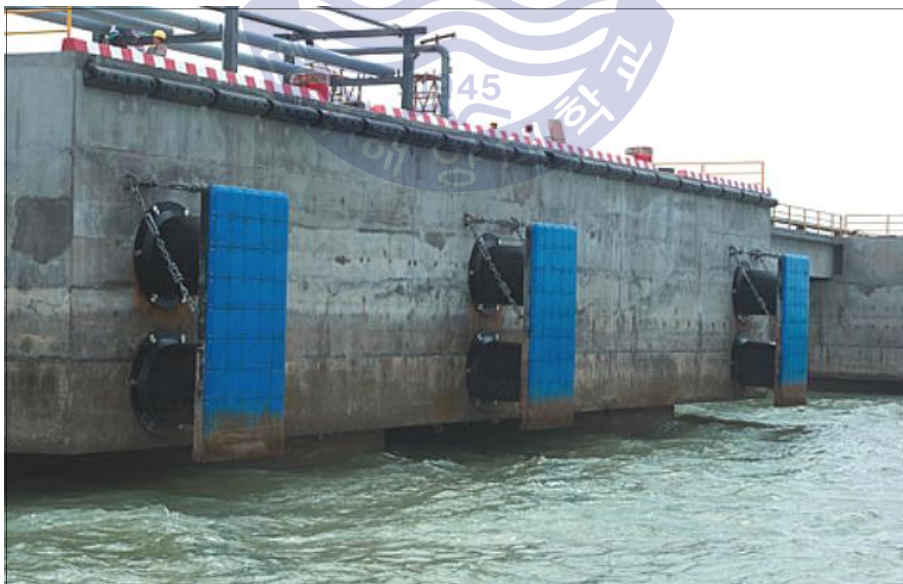
Fig. 37 Cell type fender
