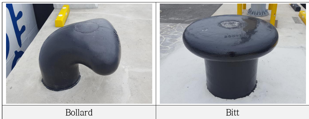
Fig. 93 Bollard and bitt in the Busan international passenger terminal
