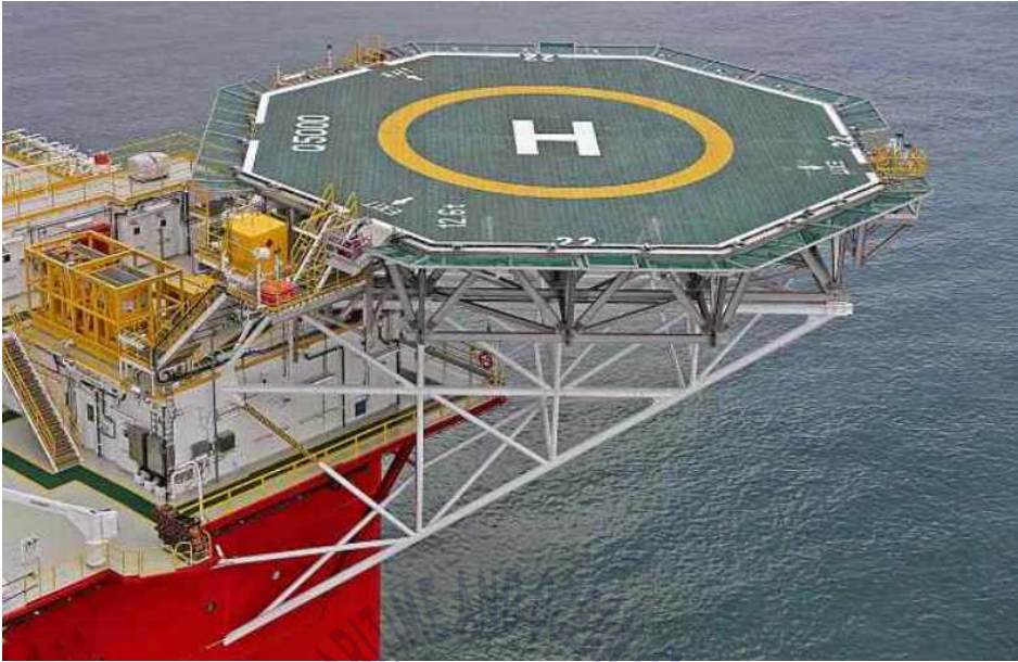
Fig. 1 Aluminum alloy helideck on offshore platforms
