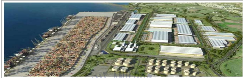
자료: Adams Hendry, http://www.adamshendry.co.uk/london-gateway-ldo
