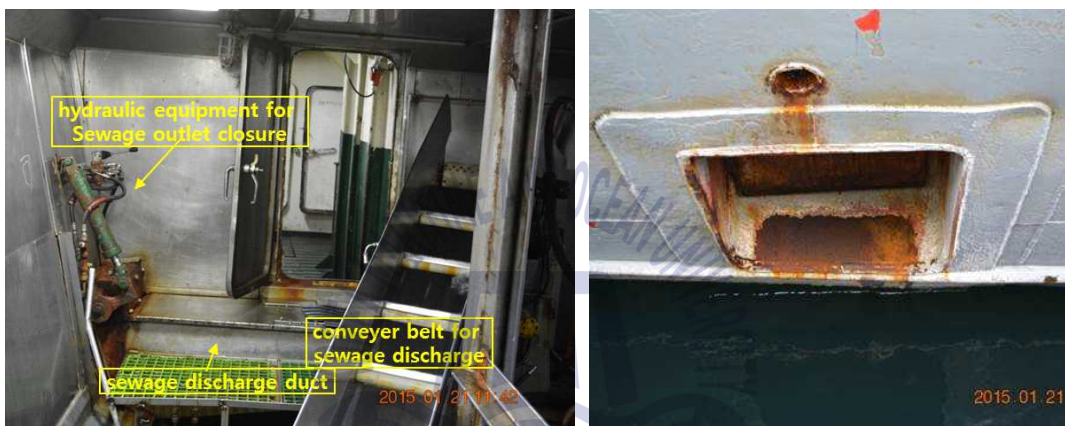
(e) inboard and outside scenery of sewage outlet
