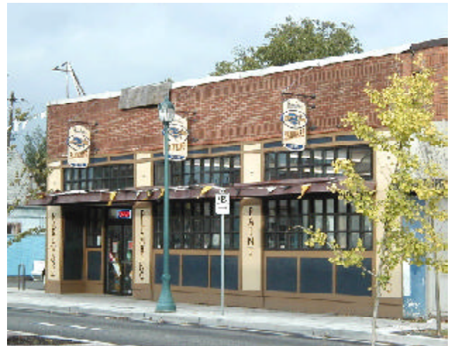
Hankins Hardware Storefront Improvement
