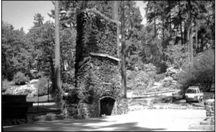
The rock fireplace in the Picnic Shelter (being restored) provides a strong sense of place.
