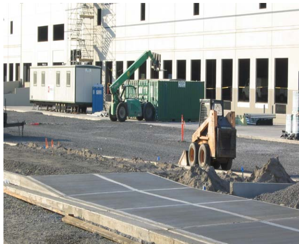
New construction in Rivergate.
