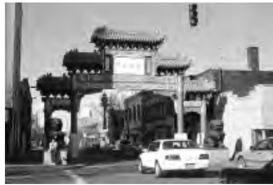
Chinatown Gate at 4th Avenue
