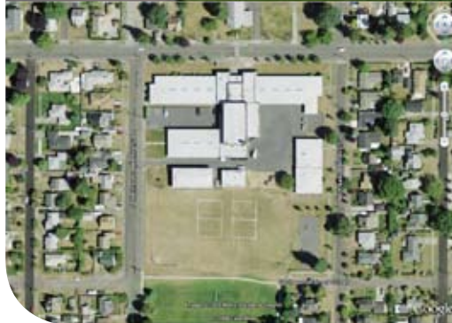
Harvey Scott School - aerial
