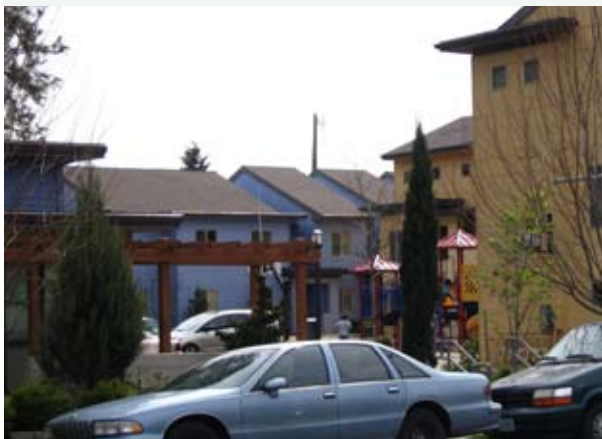
New family-oriented housing in Cully.
