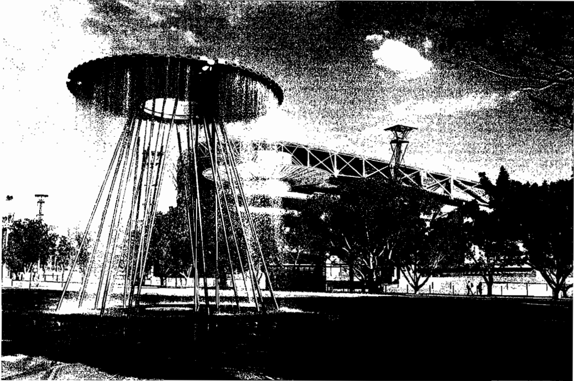
Figure 7. In the spirit of re-use, the former cauldron which held the Olympic flame throughout the 2000 Games has been modified, and now serves as a fountain. The overflow area where it stands will be in-filled with residential and commercial development as part of a 2020 Master Plan developed by SOPA. In the background is a streetlight which is powered by solar panels.
