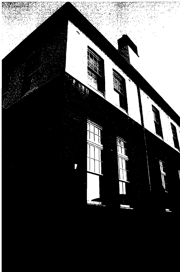
Figure 3. Building A of the Abbatoir Heritage Precinct, pictured above, acted as the administration building for the new abbatoir in Homebush Bay. Once central to the abbatoir complex, it is now situated in the heart of Sydney Olympic Park. Building A presently houses the Australian Paralympic Committee and Sport Knowledge Australia.
