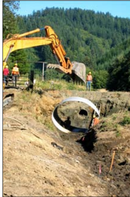
The Siuslaw Stewardship Group uses stewardship contracting to restore natural watershed processes, such as repairing or replacing culverts for safe fish passage.
