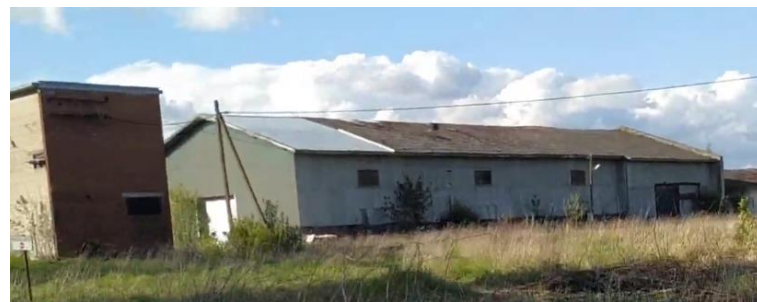
Photo nr 58. Pilka centre, old sovkhos farm complex
