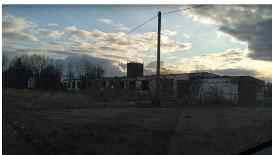
Photo nr 27. Old luunja sovkhov farm structures, abandoned
