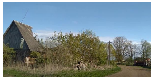
Photo nr 50. „Sahkapuu“ school location, old farm complex, in a bad condition (2)
