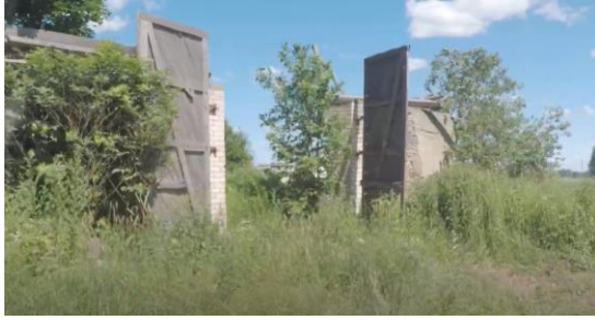
Photo nr 8. „Sahkapuu“ school location, old farm complex (2)
