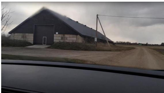
Photo nr 28. Old Luunja sovkhos farm structure, located at “Ringraja”, restructured for modern use
