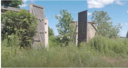
Photo nr 8. „Sahkapuu“ school location, old farm complex (2)
