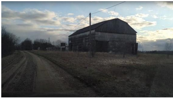
Photo nr 31. Luunja sovkhov farm buildings, old stable, abandoned looking
