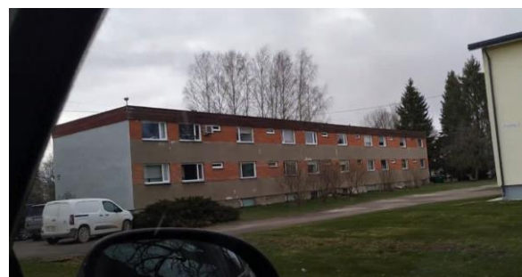
Photo nr 37. Luunja centre, sovkhos era apartment building
