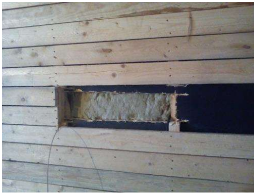
Figure 3. Applying sensors between layers.
