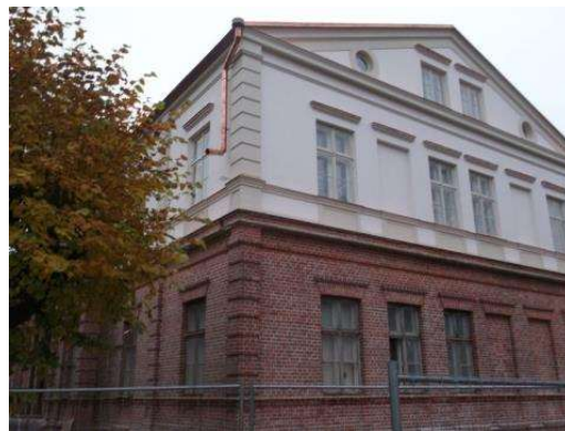
Figure 2. Veski 13 after renovation.
