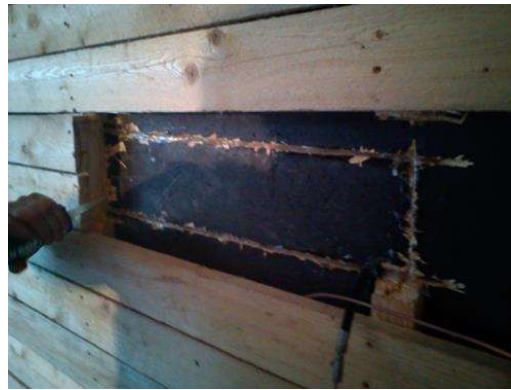
Figure 4. Sealing the opening with silicone.
