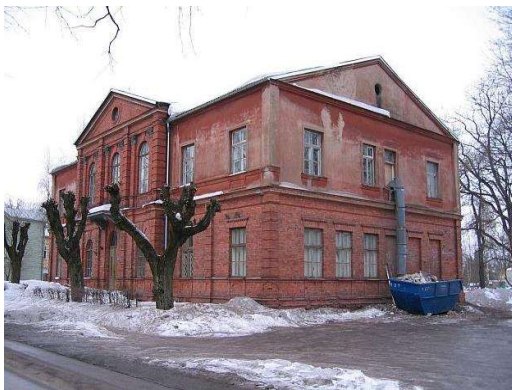
Figure 1. Veski 13 before renovation.
