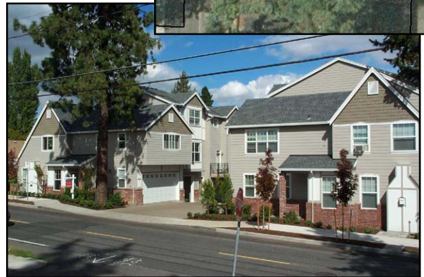
Townhouse cluster with central driveway, Southwest Portland. General configuration is similar to what would be facilitated by the shared street concept. In contrast to typical rowhouse projects, curb cuts are minimized and end units reflect the massing of detached houses.
