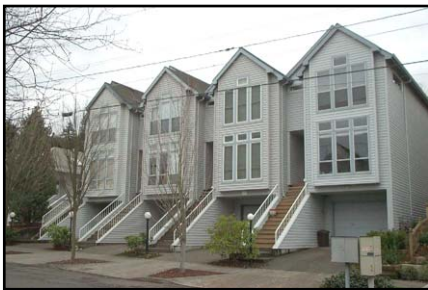
Rowhouses typical of infill in the 1980s and 1990s.
