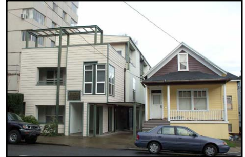
Three-story fourplex, with top floor set back.
