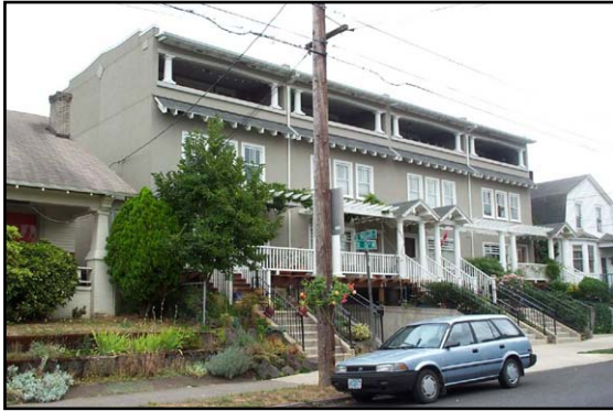
Four-level rowhouses whose height is broken up by porches, recessed balconies, and by partially excavated parking.
