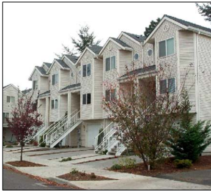
Below: Recent rowhouse, plex, and apartment projects with frontages dominated by vehicle facilities.
