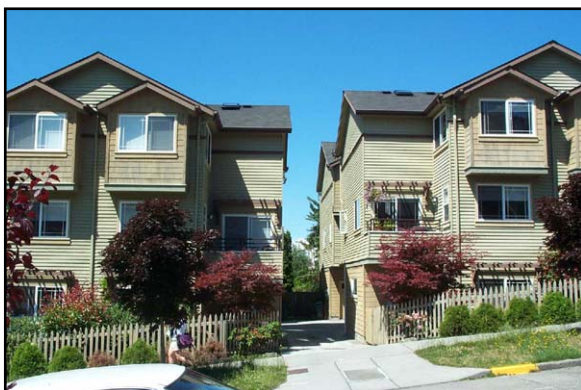
10.5' driveway serving 8 townhouse units
