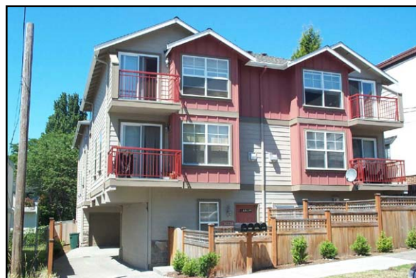
10.5' driveway serving 4 townhouse units
