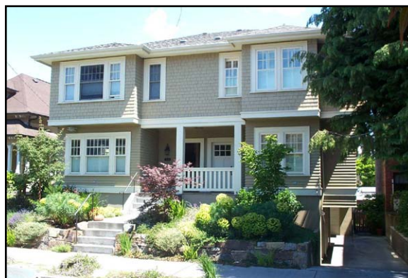
11' driveway serving 4 townhouse units
