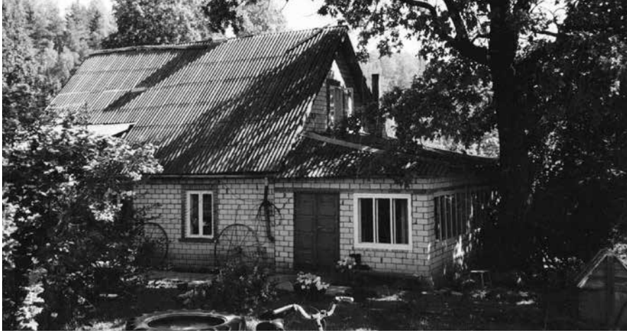
Fig. 5. The structural logs of the residential building at the farmstead of Sibula 2 originate from a log structure in the farm of the mother of the current owner of the Sibula 2 farmstead. They were brought to Sibula 2 in 1956, where they were reassembled and sided with silicate bricks, a highly popular construction material of the Soviet period. (Photo: P.-K. Parts)
