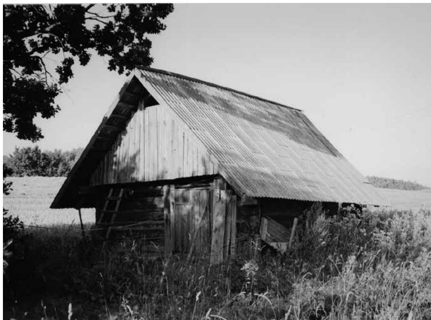
Fig. 1. A smoke sauna at Püssa farmstead, probably built in the beginning of the 20th century. Saunas in Estonia started to be equipped with chimneys at the end of the 19th century. The original smoke sauna tradition has persisted mainly in the outlying regions, including the territory of the Karula National Park. Because of the fire hazard they represented, saunas were usually constructed at a distance to other buildings. (Photo: P.-K. Parts)
