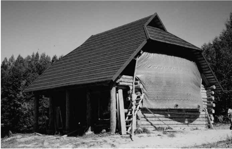
Fig. 3. The combined sauna/summerhouse at Pihlemäe (still in the process of construction in 2002 when this picture was taken) fits harmoniously into the discourse on the building traditions in Karula. Old smoke saunas in general tend to have a slim look – built of hewn logs, the height of their gable-end, as a rule, slightly exceeds their width (see Figure 1). They are usually located in a low spot, away from other structures, and evoke a parallel to a poor relation shunned by the main family. The ‘traditional saunas’ constructed at the turn of the millennium tend to be built of unhewn logs, using the (allegedly) ancient round-notch corner and leaving the overhangs to jut out at varying lengths. This is no longer a poor relation – we are looking at an architectural showpiece. (Photo: P.-K. Parts)
