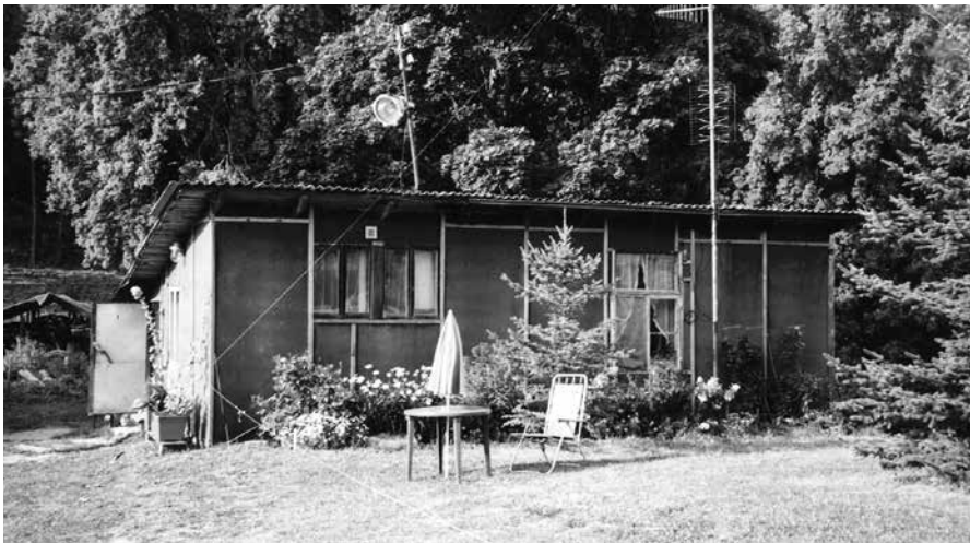
Fig. 6. The cabin at Soesaare was built in the 1990s on a surge of euphoria that characterised the period when Estonia regained its independence and many family farms were re-established. It is somewhat difficult to situate this structure in the discourse on ‘the building traditions in Karula’. Yet, at the time this photograph was taken (2002) it served as the dwelling house / milk cooling facility for Karula’s last dairy cattle farmer who kept a considerable tract of land clear as pasture and, in so doing, effectively contributed to maintaining semi-open semi-natural ‘national landscapes’ – a priority protection goal of the Karula National Park. The structure served its residents for ten years, effectively functioning as an initial foothold that made it possible to maintain traditional land use and eventually to construct a ‘more sophisticated’ dwelling. (Photo: P.-K. Parts)
