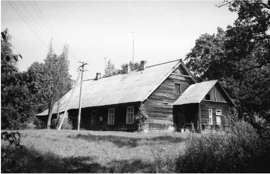
Fig. 4. There is little doubt that the dwelling house at Mäe-Mähkli (built in 1928) represents an instance of traditional architecture of Karula, although it does not belong to the oldest period from which specimens have been preserved – that of the 19th century barn-dwellings. The barn-dwelling is a type of farm dwelling unique to Estonia and North Latvia. Its particular feature is the fact that it had a double function – barn-dwellings were used both as a residence and as an agricultural production facility (for crop drying, threshing, etc.). The corresponding structural peculiarity of preserved barn dwellings is in most cases difficult to recognise because of repeated remodelling and various subsequent extensions, the aim of which was to give the barn-dwelling the appearance of more modern dwelling houses. (Photo: P.-K. Parts)
