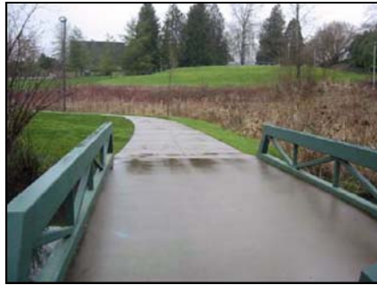
Figure 3. Concrete Trail in Stream Corridor
