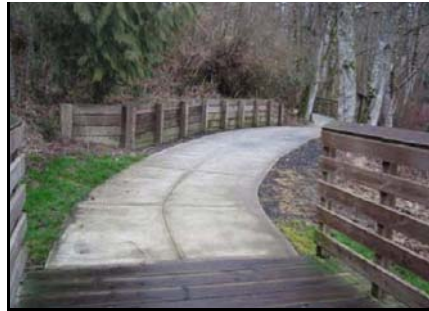
Figure 5. Concrete Trail Transitions to a Boardwalk
