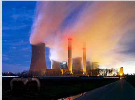
Scrubbing and supply of CO 2
