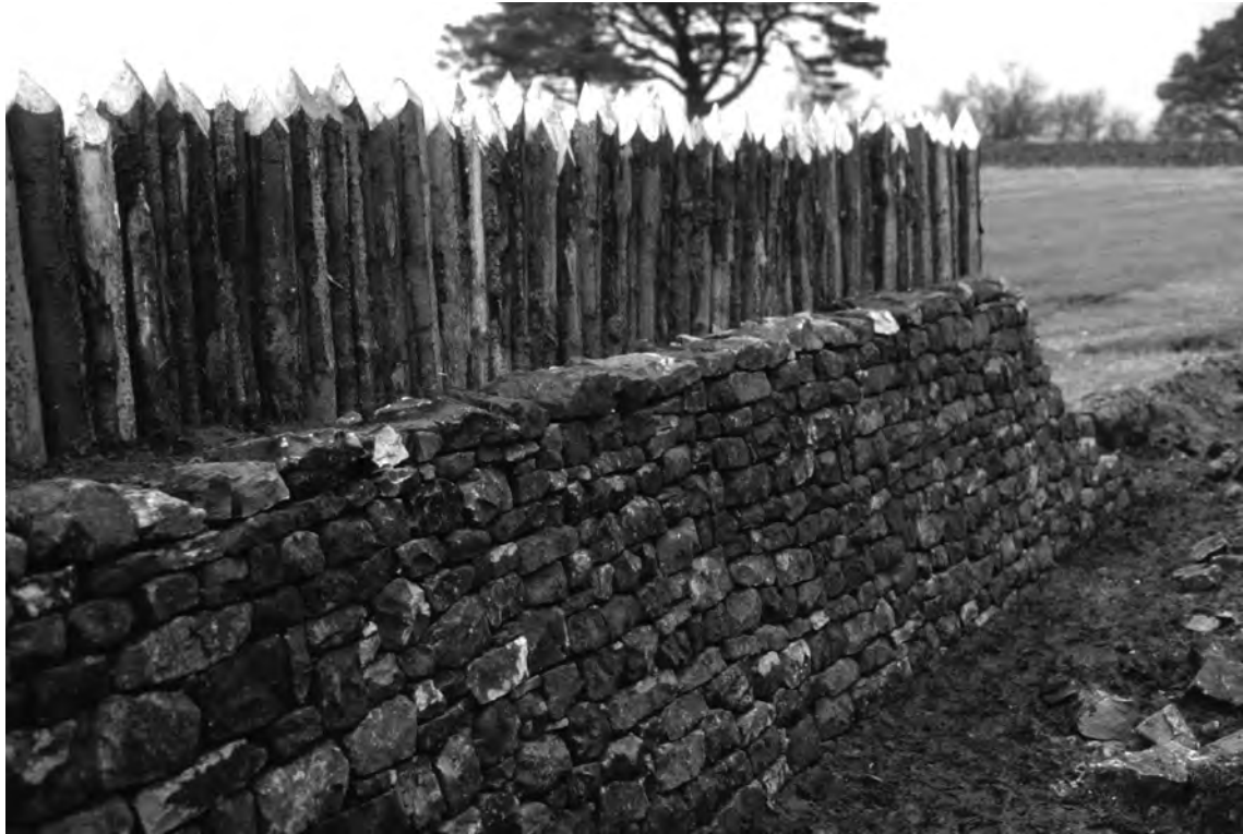
Fig. 5.42. The experimental reconstruction of dry-stone walls at Brigantium, reaching at least 2.5m in height with space for a heavy timber breastwork set in clay, based on the width of the wall bases observed during the excavations at the nearby site at Woolaw.
