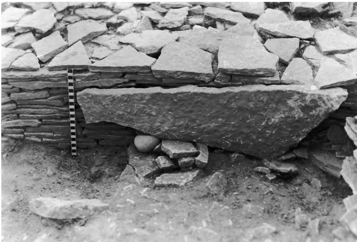
Fig. 4.62 The outer wall on the north side of the barrow in cutting DV, opposite bay 10, from the north. Other fallen stone has been removed, revealing a large stone pitched on edge against the outer wall. Compare Fig. 4.63, the same stretch at an earlier stage of excavation.
