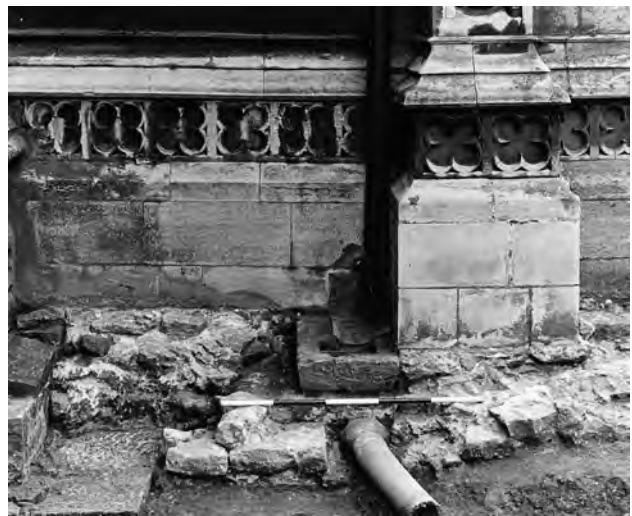
Fig 2.36 Looking west at the foundations cg103 of the Fleming Chapel: lc84 Area A, LUB 2
