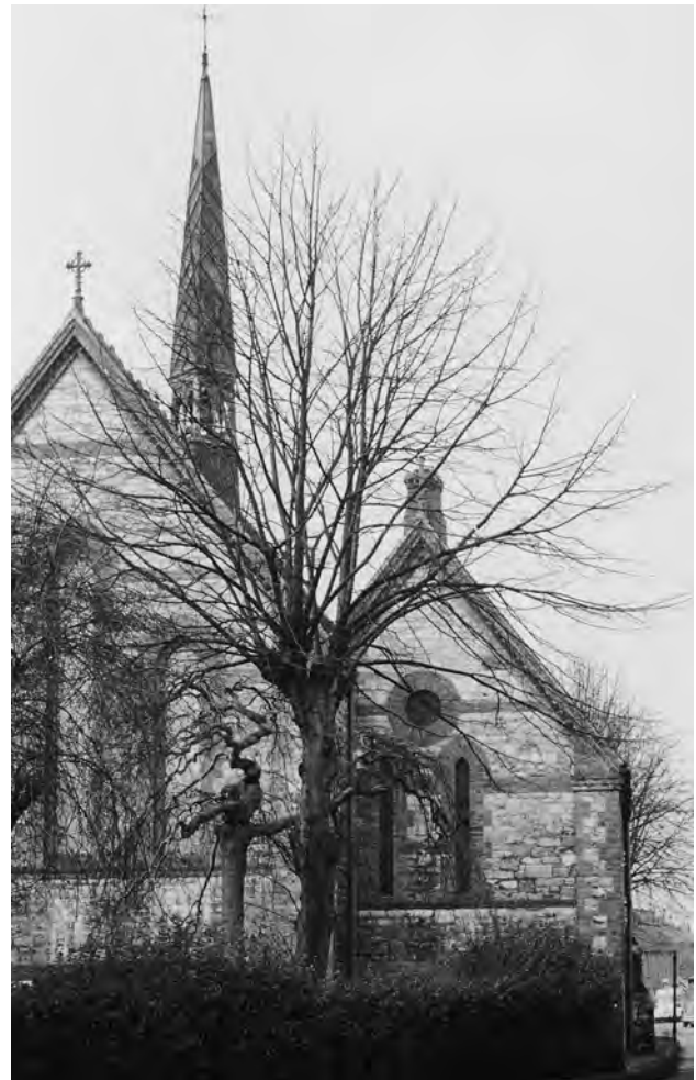
Fig 9.51 View of the Victorian church from the east, shortly before its demolition in 1970
