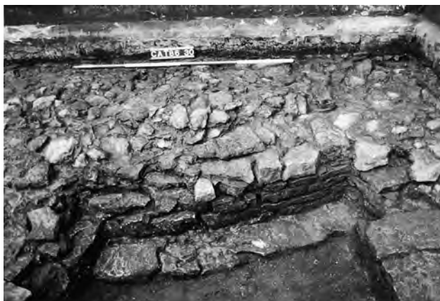
Fig 2.40 Looking south at the foundations cg6 of one of the radiating chapels of St Hugh's Choir; the foundations are abutted by later wall cg21, which can be seen (right); the foundations cg36 of the Angel Choir were built over cg6: cat86, LUBs 10, 11, and 14
