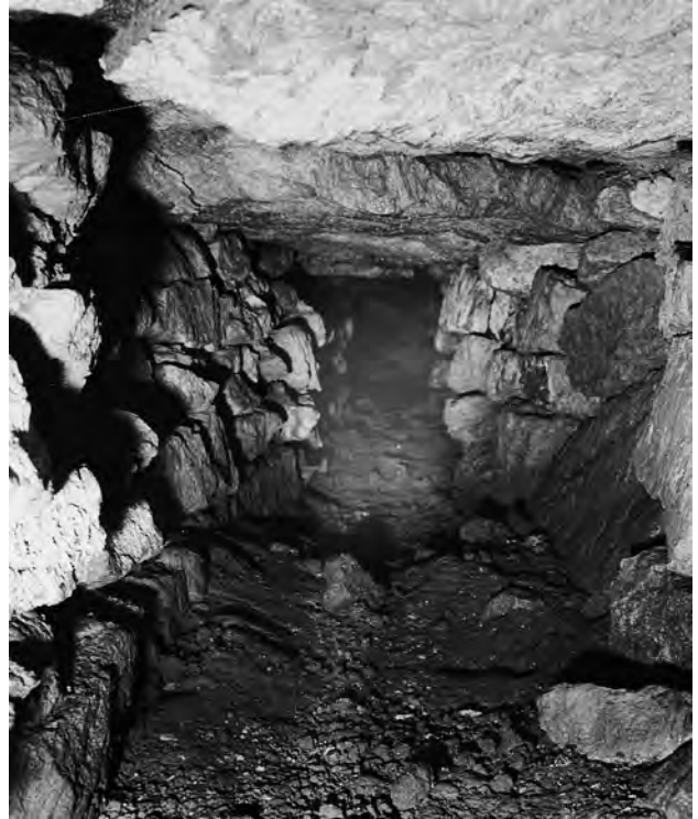
Fig 5.16 Looking east inside the drain cg34: LUB 13
