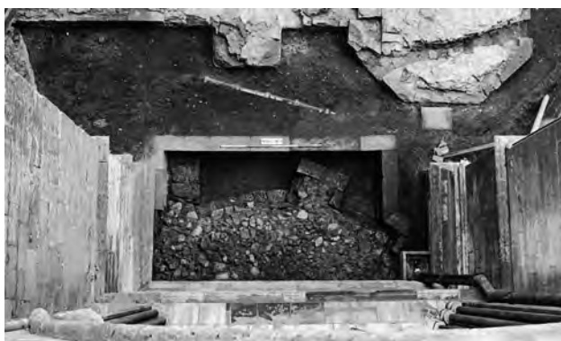
Fig 2.41 Looking down the walls of the Angel Choir cg36, facing north on the foundations cg6 of one of the radiating chapels of St Hugh's Choir; to the north-west the chapel is abutted by a north-south wall cg12; the chapel foundations are encased by wall cg21; the chapel foundations cg7 can be seen to the north: cat86, LUBs 10, 11, 12, 14 and 22
