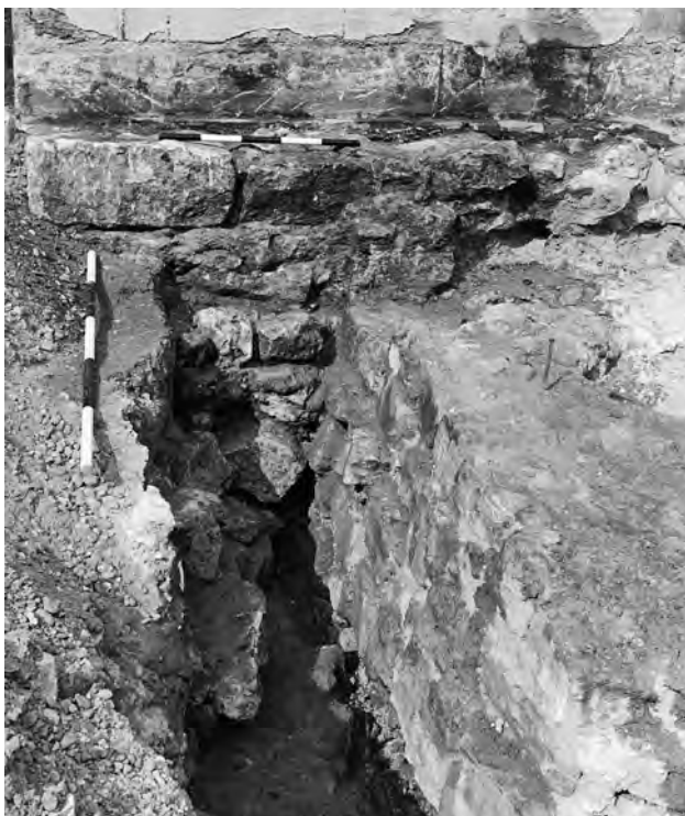
Fig 2.44 Looking north-east at the west side of the east wall cg201 of the upper colonia, reused to underpin the foundations cg229 of St Hugh's Choir: lc84 Area B, LUBs 25 and 26
