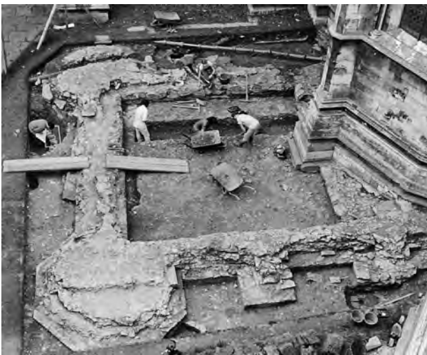
Fig 2.34 Looking south giving a general view of cat86 under excavation
