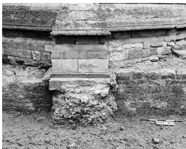
Fig 2.38 Looking west at the east face of the west wall cg4 of the Roman/Norman defences; sealing the truncated wall were the foundations cg7 of the chapel and over the levelled remains of these, the 1773 chapel cg23: cat86, LUBs 9, 12 and 20
