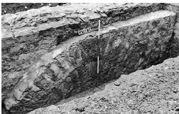
Fig 2.42 Looking south-east at the relieving arch in the foundations cg32; foundations cg7 were constructed above: cat86, LUB 12
