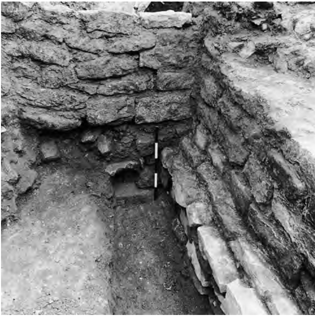
Fig 12.19 Looking east at Structure 3.3; wall cg9 with hole for drain cg91: LUB 5
