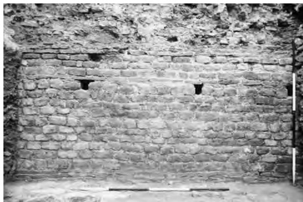
Fig 12.28 North face of Mint Wall as excavated, built over Structure 1. Compare small stone blockwork to Figs 12.26–27.
