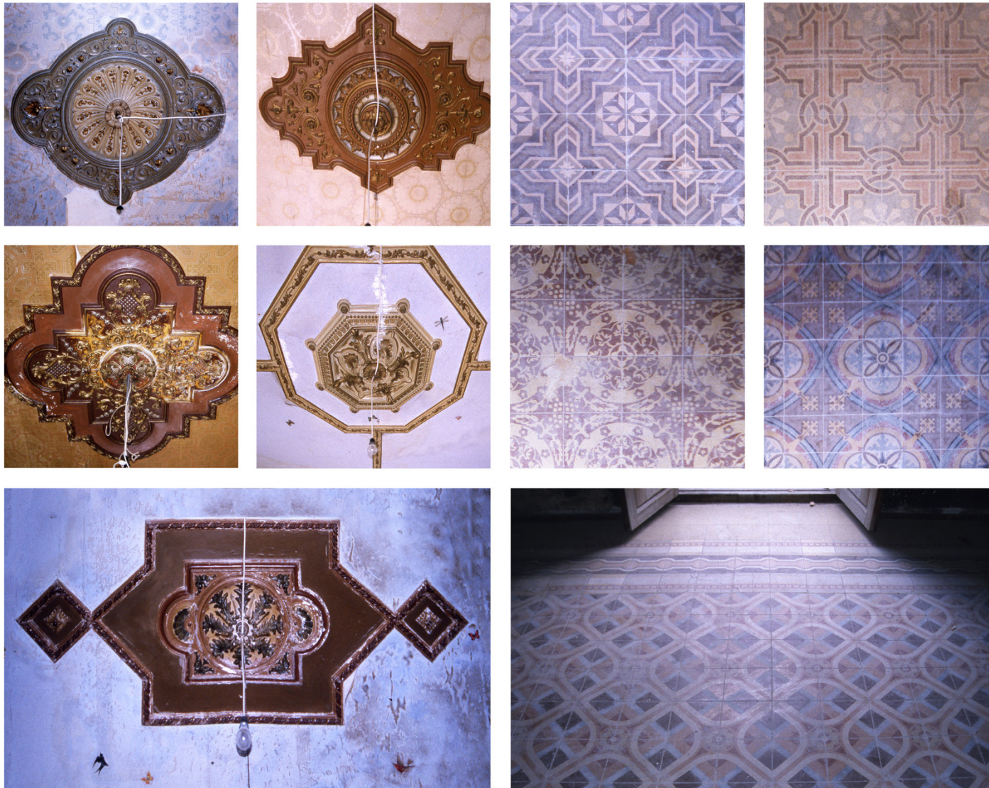
Fig. 17. Casa de l'Hort (former Residence-Palace of the Cardinal Payá), Onil (Alicante, Spain), Feb-1996. Photographies of the Initial of the Building before its Drawing and its Rehabilitation. Photographs of the finishes of the Main Floor (Noble Plan, Fig. 10); left: plaster ceiling moldings; right: flooring for hydraulic parts. (Original Pictures: Martínez-Medina, A. & Sempere Valero, M.).
