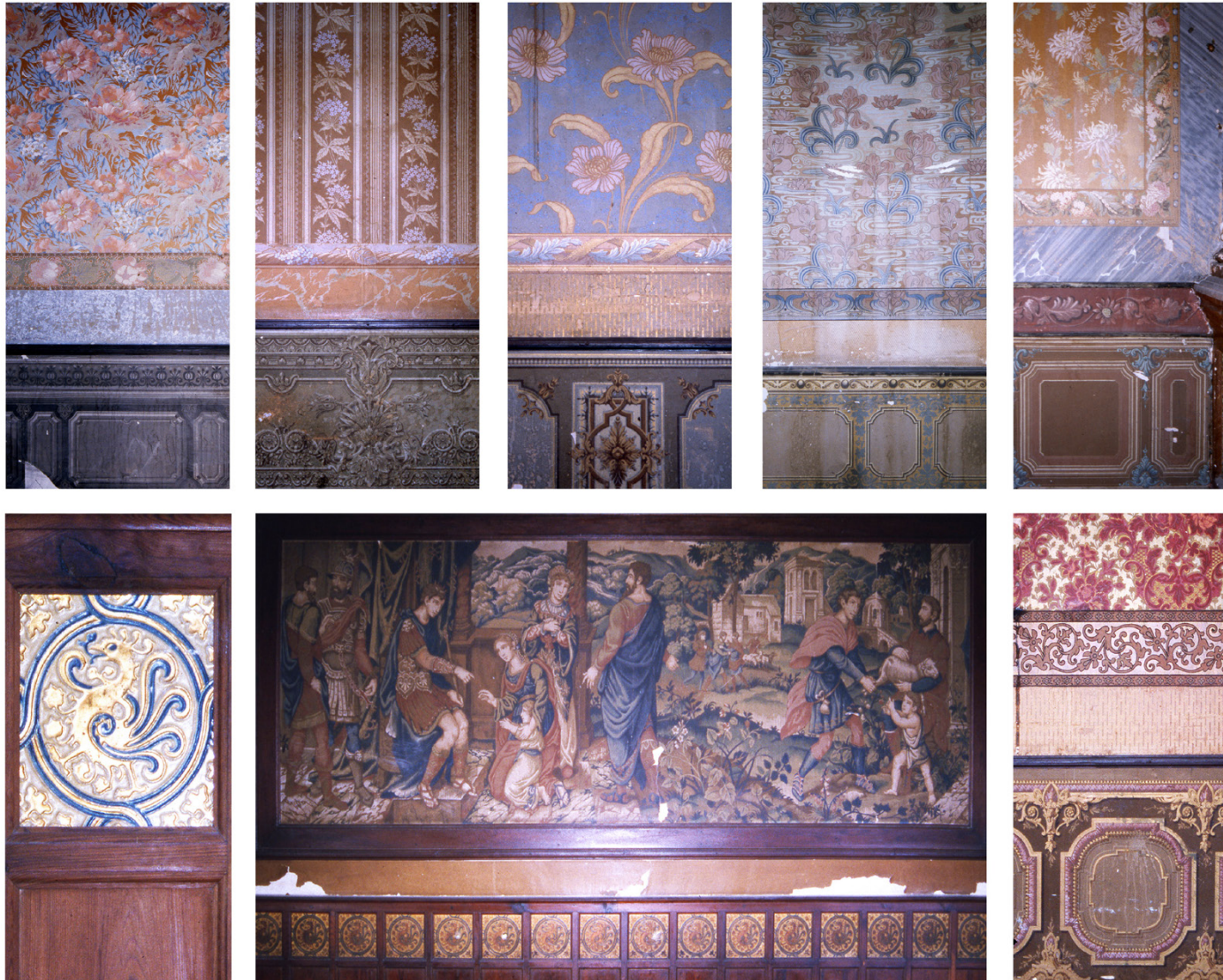
Fig 18. Casa de l'Hort (former Residence-Palace of the Cardinal Payá), Onil (Alicante, Spain), Feb-1996. Photographies of the Initial of the Building before its Drawing and its Rehabilitation. Photographs of the finishes of the noble plan (first floor); top: wallpapers on walls; bottom: wooden or ceramic plinth details. (Original Pictures: Martínez-Medina, A. & Sempere Valero, M.).
