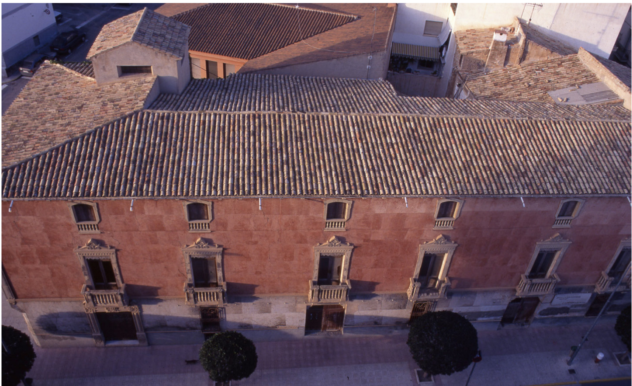
Fig. 0. Current state of the Casa de l'Hort in Onil, Palace-Residence of Cardinal Payá (Author 1996).
