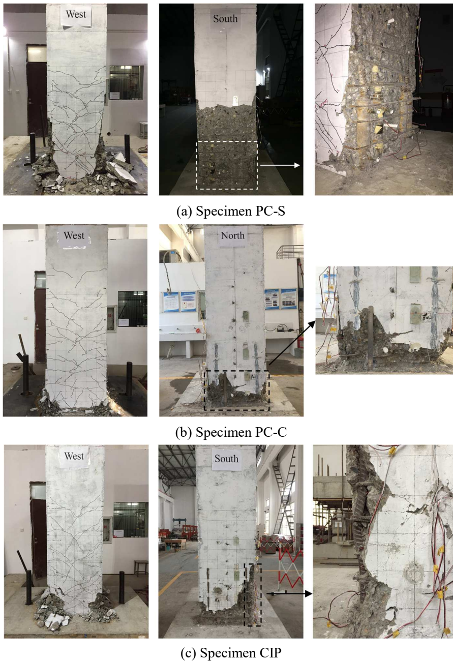
Figure 12 Crack patterns and failure modes
