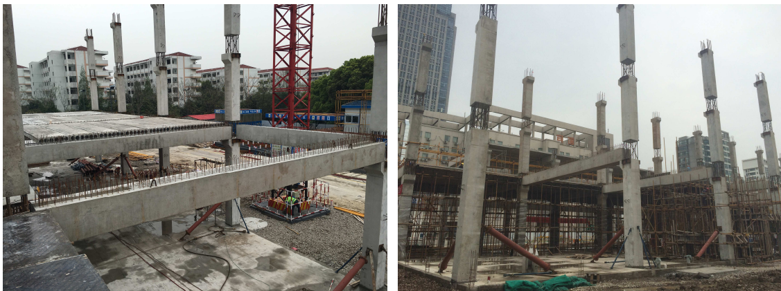
Figure 1 Multi-storey precast reinforced concrete columns
