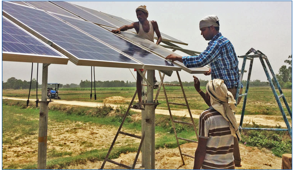
Oorja's first project in 2017, deployed to provide household electricity via a solar mini-grid, supplies clean energy to 44 households with an average of 6 to 8 family members each. While still running, Oorja's newer grids focus on serving the agricultural sector. Photo courtesy of Oorja.
