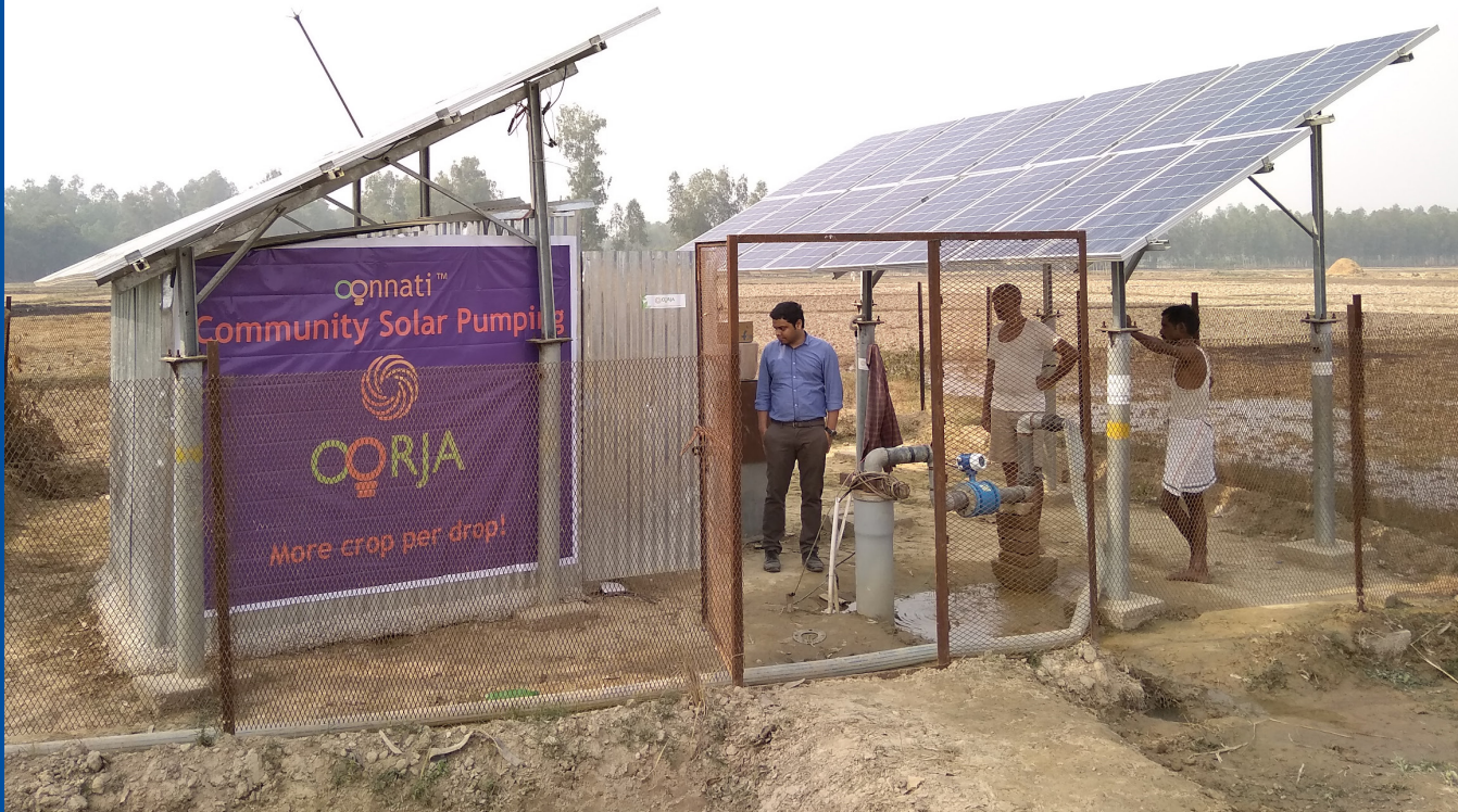
Oorja currently operates fifteen community solar pumps each of which deliver 250–320 cubic meters of irrigation water to smallholder farmers each day. Photo courtesy of Oorja.
