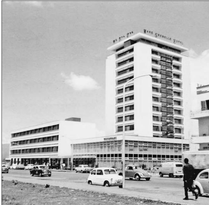
FIG. 11 B. PETROVIĆ, WABE SHEBELLE HOTEL, ADDIS ABABA, ETHIOPIA, 1968: THE BUILDING ON A HISTORICAL PHOTO (UNKNOWN DATE)
