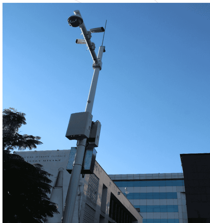
Image 2. Cameras are fixed, static, and can pan tilt and zoom (Main Mall). Photo: S. Molepo.
