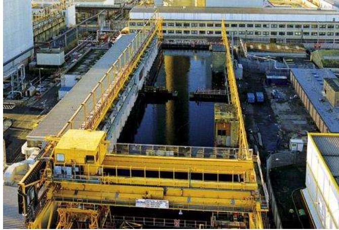
Figure 4: Pile Fuel Storage Pond (PFSP). This picture shows the top view of one of UK's legacy nuclear storage ponds. The PFSP is a 100 m by 25 m by 7 m pond comprising radioactive sludge formed from nuclear fuels and debris .
