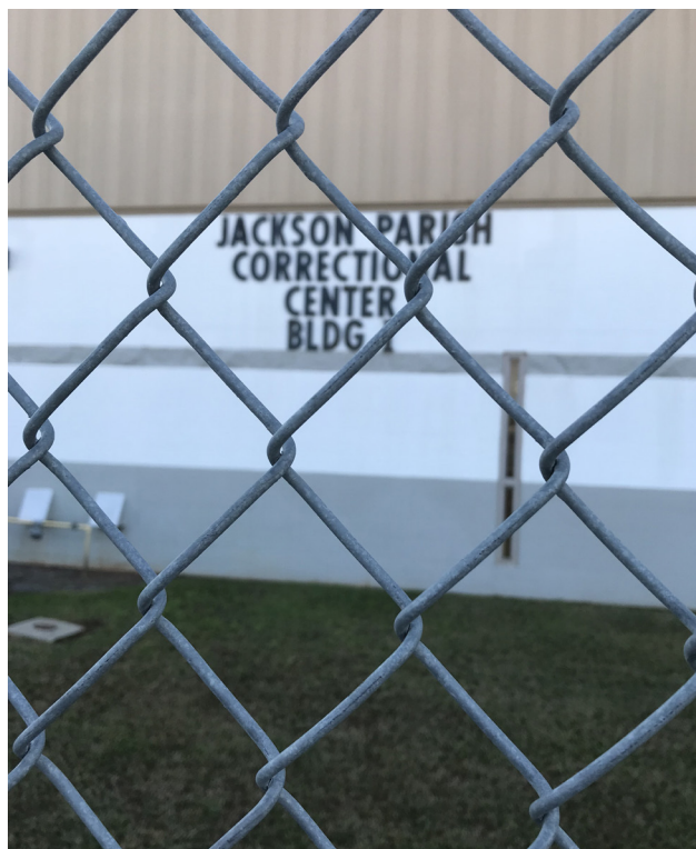
Entrance to Jackson Parish Correctional Center
