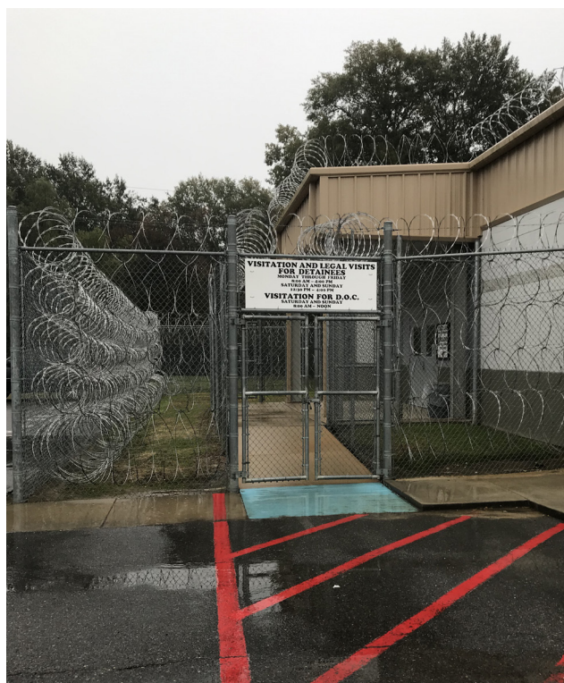
Richwood Correctional Center, Visitor's Entrance
