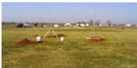
The installation of the instrumentation tower, solar panels, and weighing bucket rain gauge is completed. Solar panels help provide power to the station for the operation of instruments.
