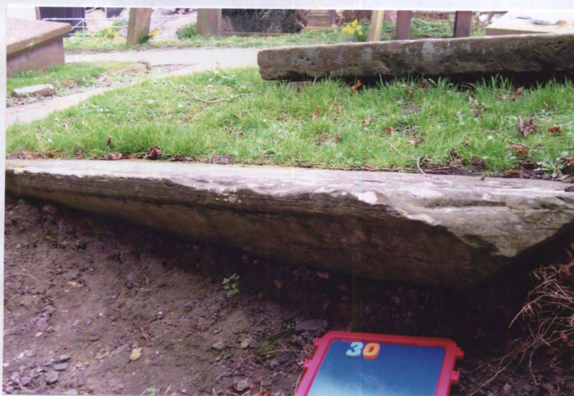
Below: Soil erosion near Memorial 30, dated c1766, reveals the peculiar subterranean tapering that may be a construction element of other ledgers within the churchyard.
