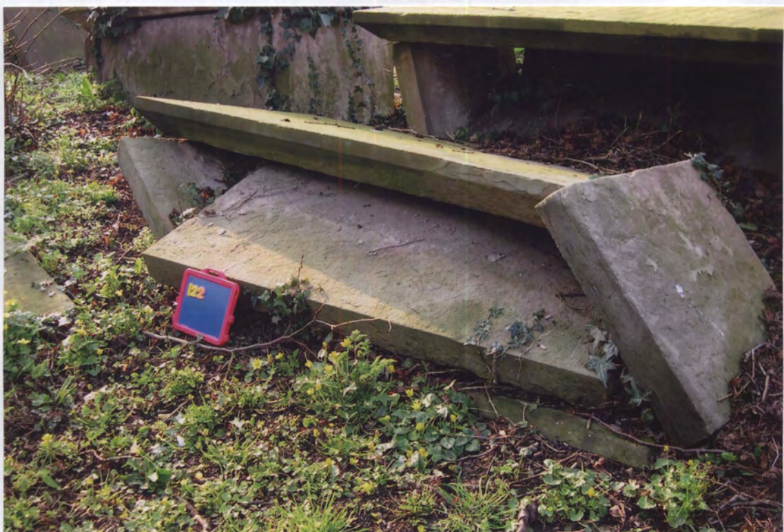
Images of decay: Memorial 129 (c. 1820) is partially submerged and beleaguered by ivy, while the complete collapse of 122 (c. 1805) provides an object lesson in the anatomy of a chest tomb.
