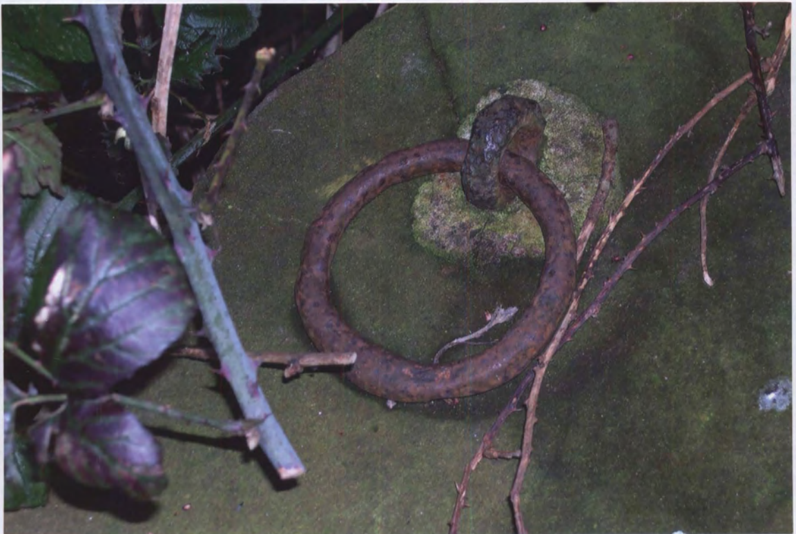
This ring on the west wall was allegedly used for mooring boats when the Dee lapped the church walls at high tide, but it bears far fewer signs of corrosion than one would expect to find in iron exposed to centuries of tidal water. An alternative theory is that some of the stones used for the churchyard wall were demolition salvage from Shotwick Castle, which once had its own quay. It may, less romantically, have been used for tethering livestock on the reclaimed pasture.
