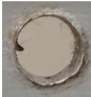
Figure 9: Hole developed on the plate after successful perforation
