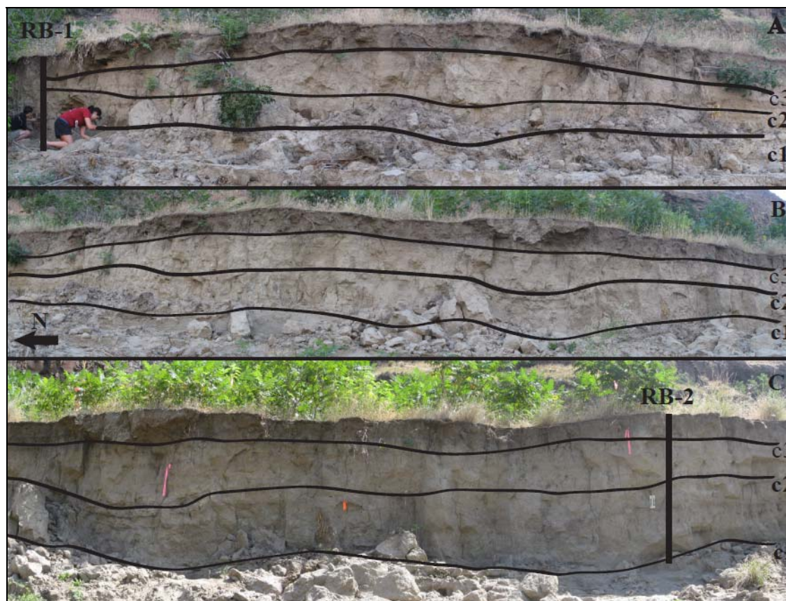
Figure 6. Photographs of the Snake River terrace cut bank. Highlighted profiles RB-1 (photo A) and RB-2 (photo C). The distance between RB-1 and RB-2 is 28 m (photo B). The black lines mark the approximate locations of three horizons containing cultural materials: c1, ~1500-1700 B.P.; c2, ~1000 B.P.; c3, ~600-700 B.P. Note: the photographs are not the same scale and overlap does occur between photos A/B and B/C.
