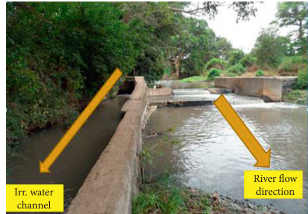
FIGURE 6: Furrow intake with no river training.
