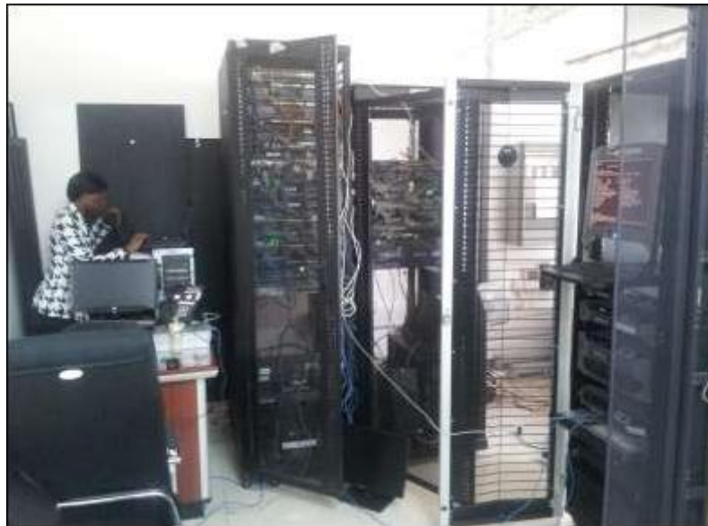
Figure 51: Performing Installation of the Model into the Server
