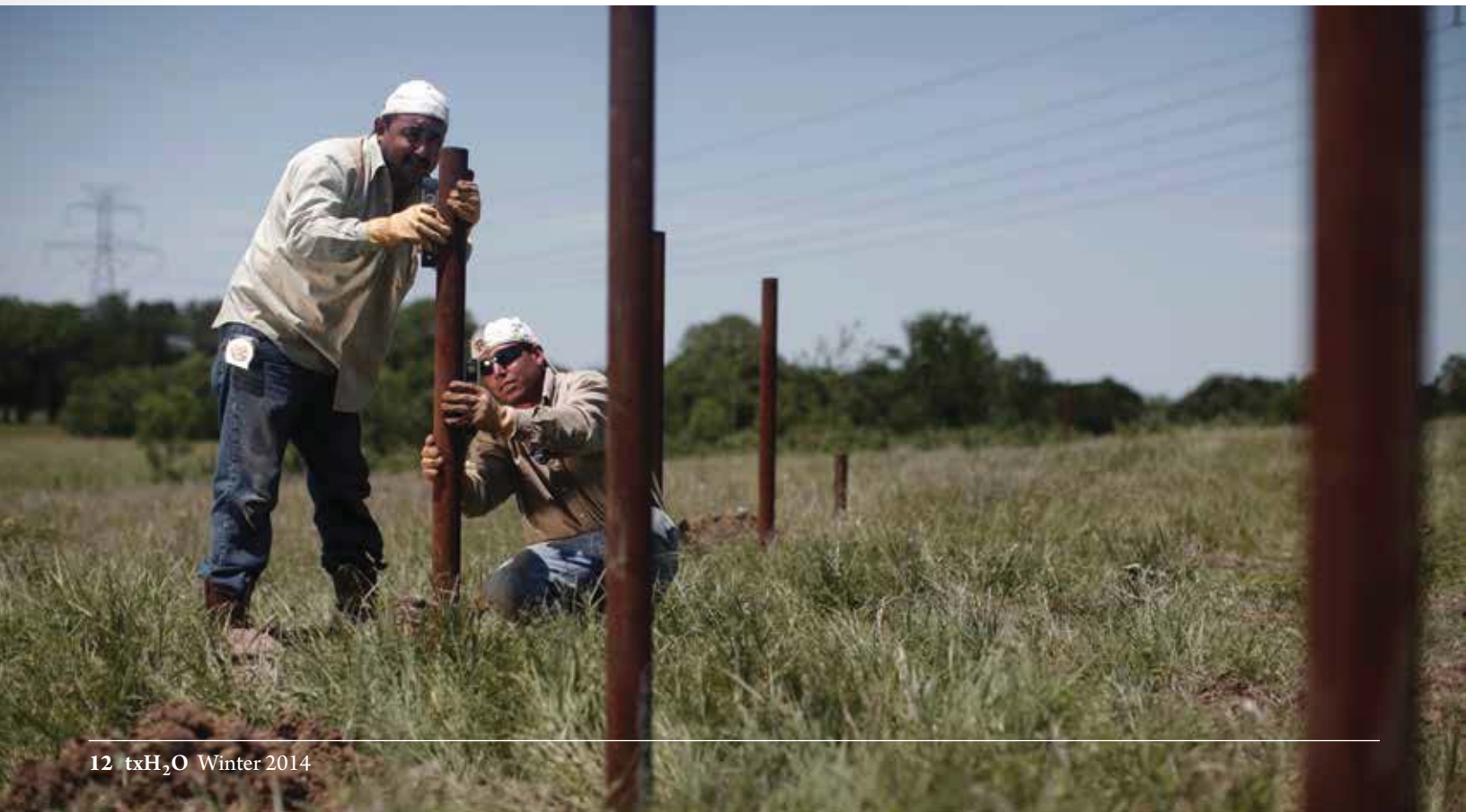
Workers install a fence on the 77 Ranch as part of Water As A Crop’s cost-share program to promote sustainable land management. Photo by Craig Ficenec, Water As A Crop.
