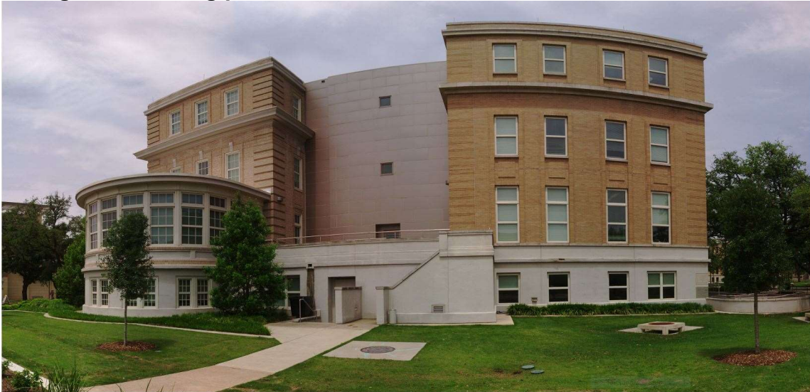
Figure 4.4 – View of the southeast facade of the Y.M.C.A. Building showing trees close to footprint of the building, captured by the FARO Focus S 350 during the scanning process.
