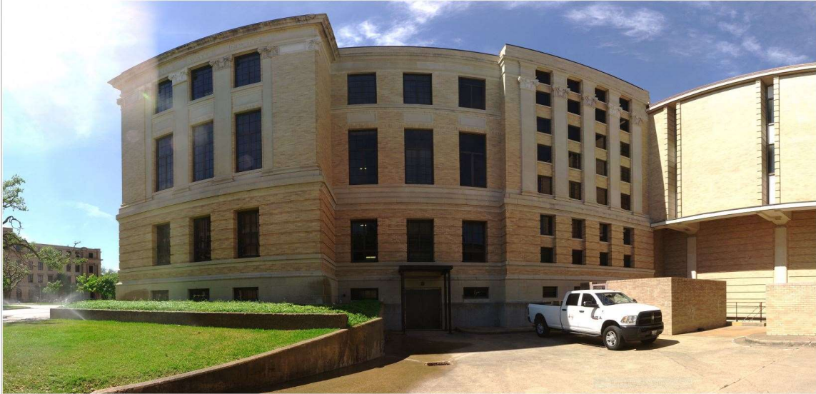
Figure 4.2 – Parked vehicle and active sprinklers on the southeast facade of Cushing Memorial Library during the data gathering process, captured by the FARO Focus S 350 during the scanning process.
