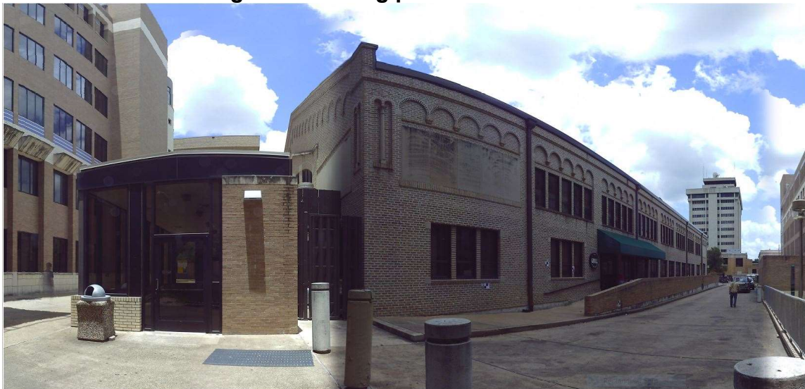
Figure 4.3 – Retaining wall for elevated walkway blocking the lower portion of the southeast facade of the Animal Husbandry Building, captured by the FARO Focus3D during the scanning process.
