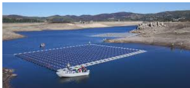
Figure 2.27 – Floatovoltaics project taking place in Northern Portugal covering 2500m 2 . Source – International Hydropower Association 2020
