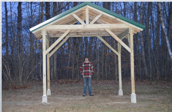
Ben LaFlamme's completed Pavilion Eagle Scout Project at Durham River Park
