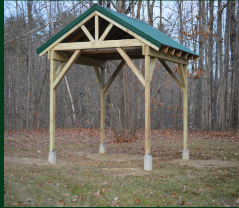
Ben LaFlamme's completed Pavilion Eagle Scout Project at Durham River Park
