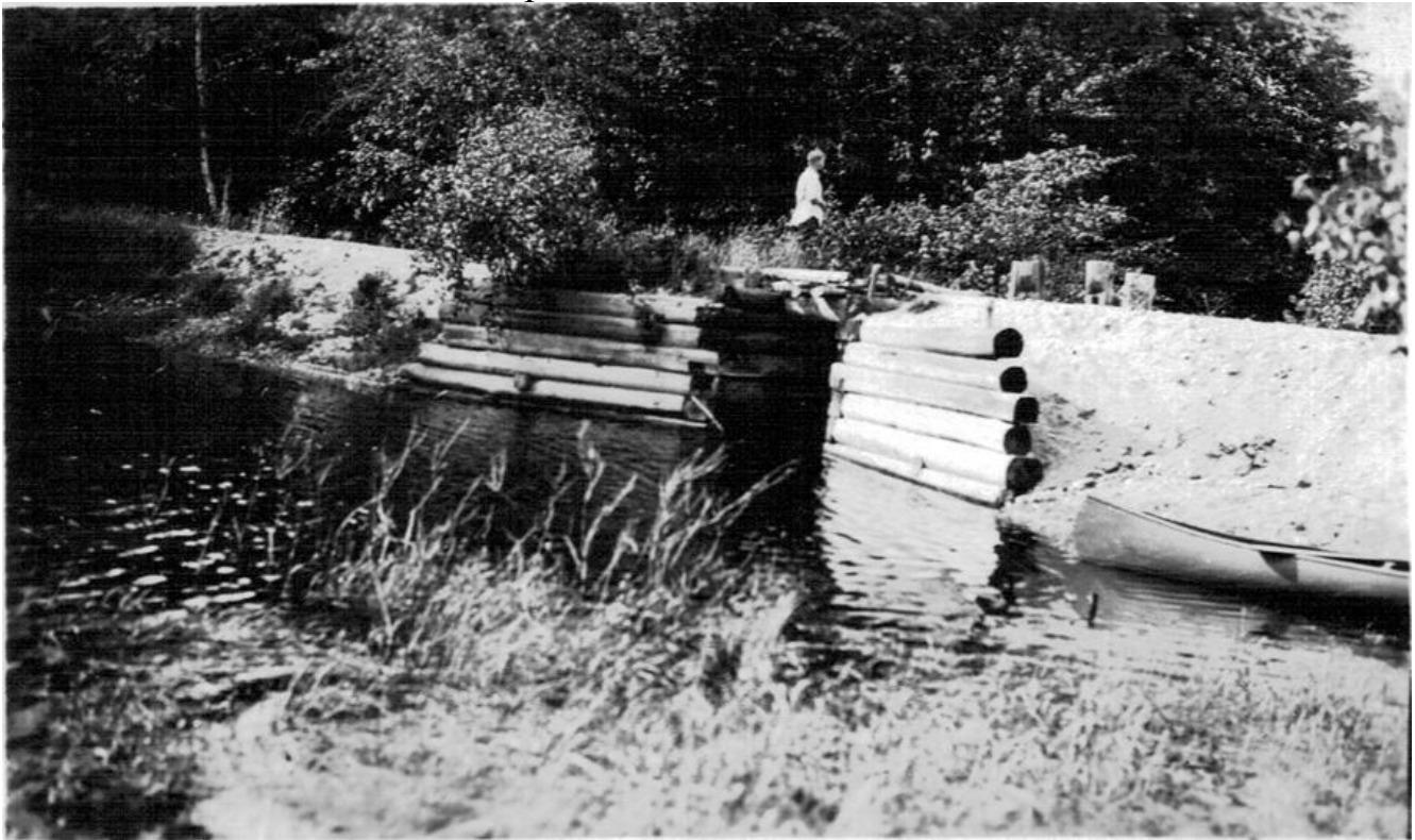
Dam on Upper Cranberry Lake – TWP 30 ca 1930
