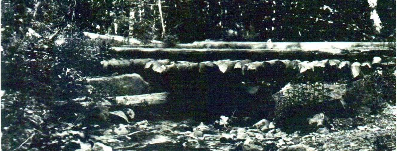
TWP 29 – Airline Road bridge over Canoe Brook – June 1924
