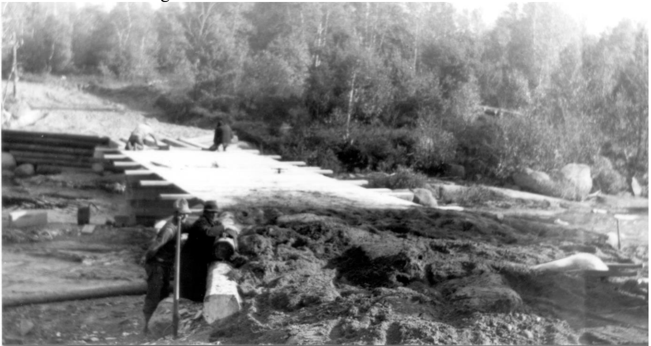
Machias River Bridge TWP 31 – Airline Road
