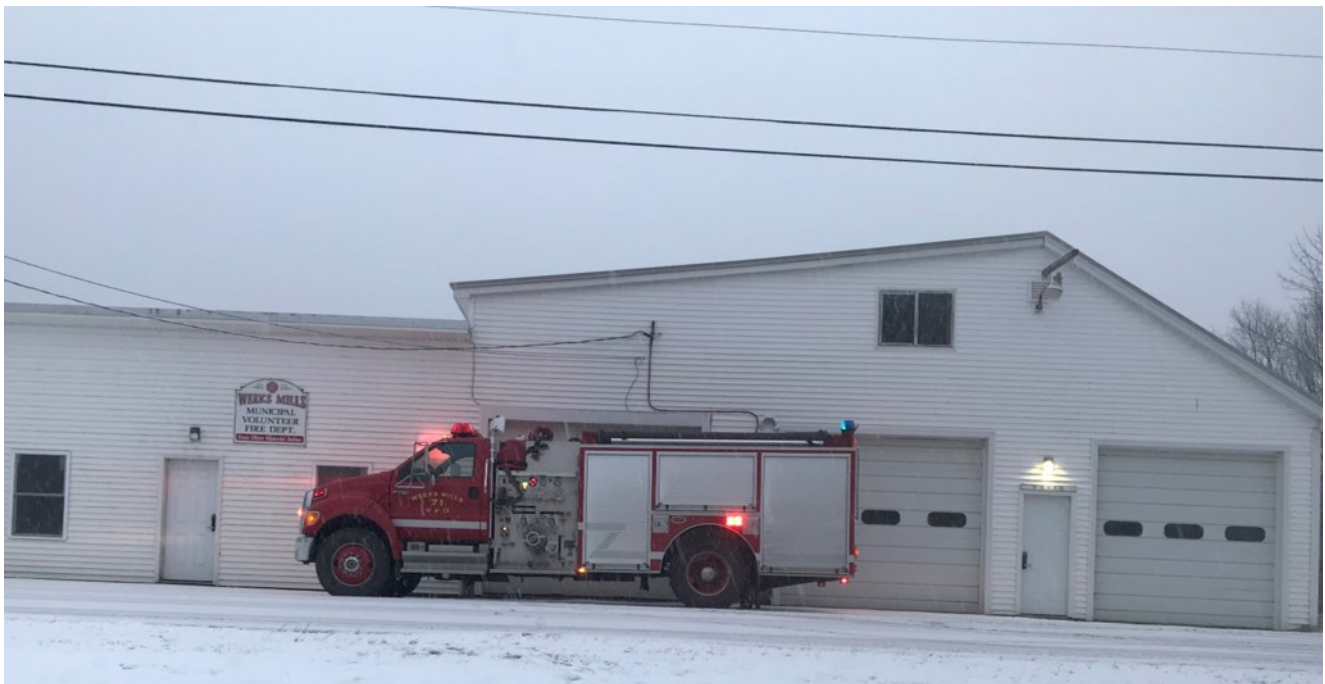
Weeks Mills Volunteer Fire Department Station
