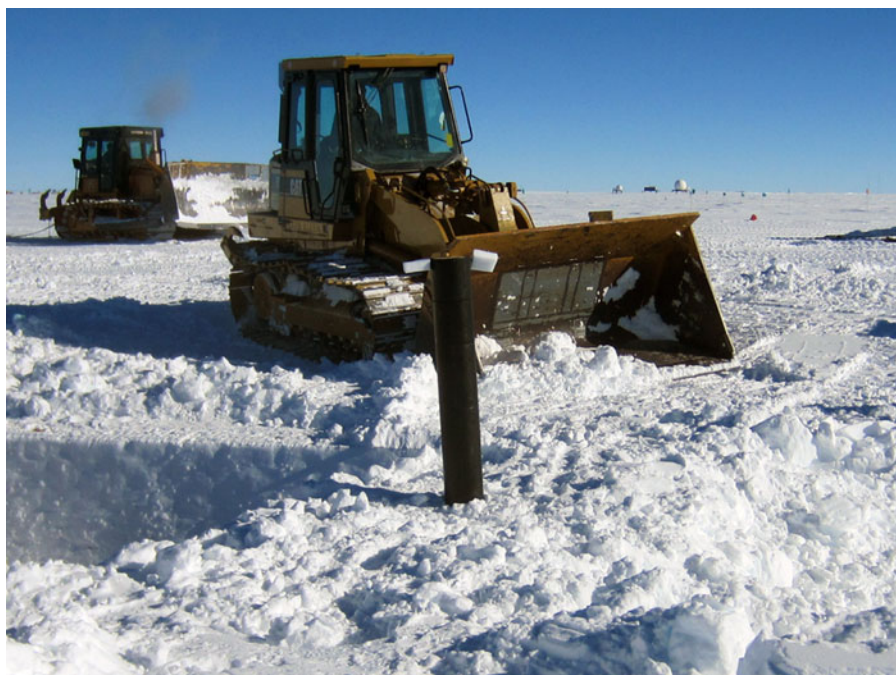
Fig. 10. At the conclusion of the project, the drill trench, drill slot and core storage trench were backfilled with snow. The borehole casing (image center) was extended ~1.22 m (4 ft) above the snow surface and the drill fluid was left in the borehole to facilitate future borehole logging or sampling.
