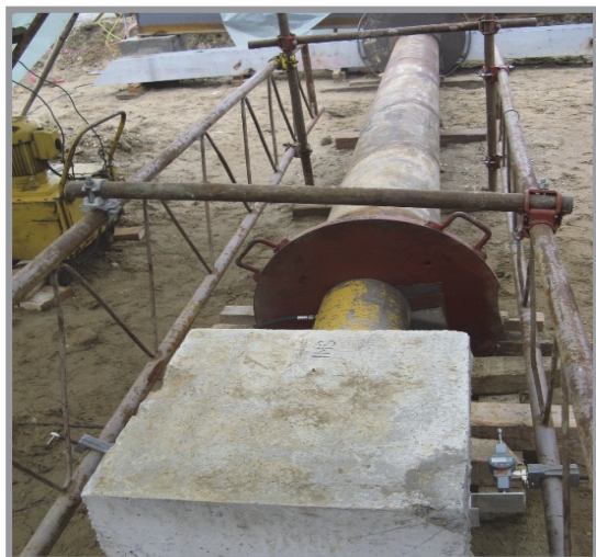
Figure 7 Setup of the pile load test for horizontal load
