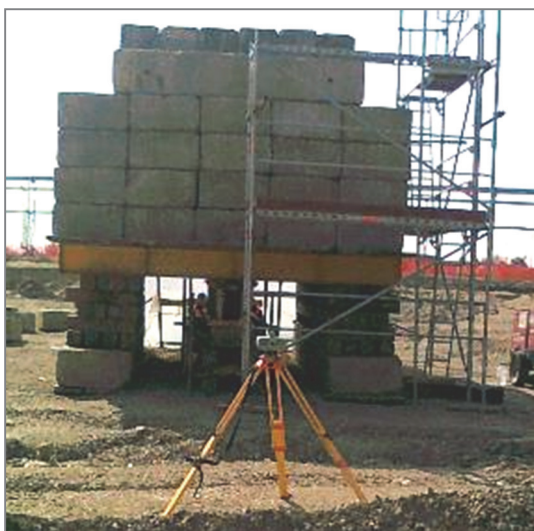
Figure 1 Setup of the pile load test for compression load
