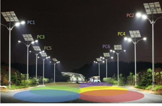
Fig.3. The illustrative scenario of the 5G coverage area using the proposed PC base station.
