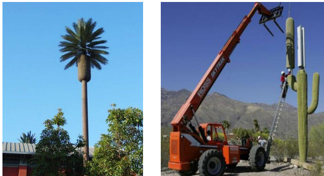
Fig.1. Base station antennas on camouflage platforms.
