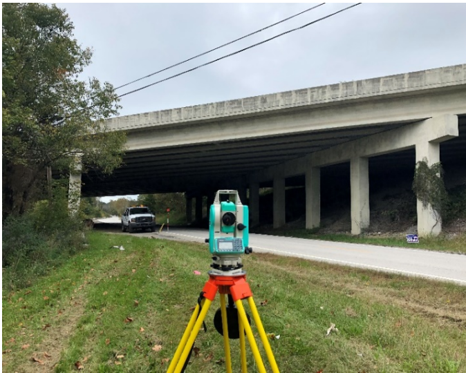
Figure 25. Total station setup.
