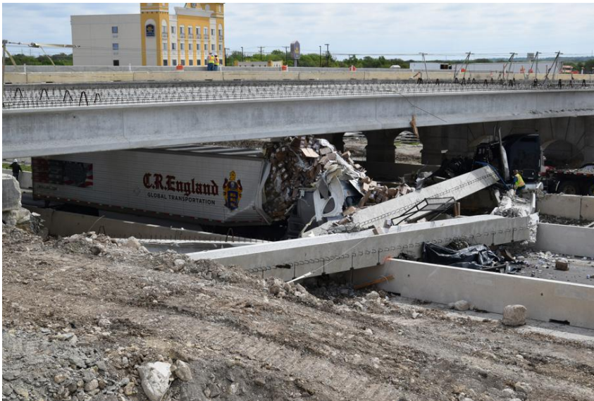
Figure 13. Salado, Texas overpass impact. Retrieved from: http://www.statesman.com/news/local/bridge-collapse-near-salado/JxaB1MxnFqOYjcDGxng6MK/
