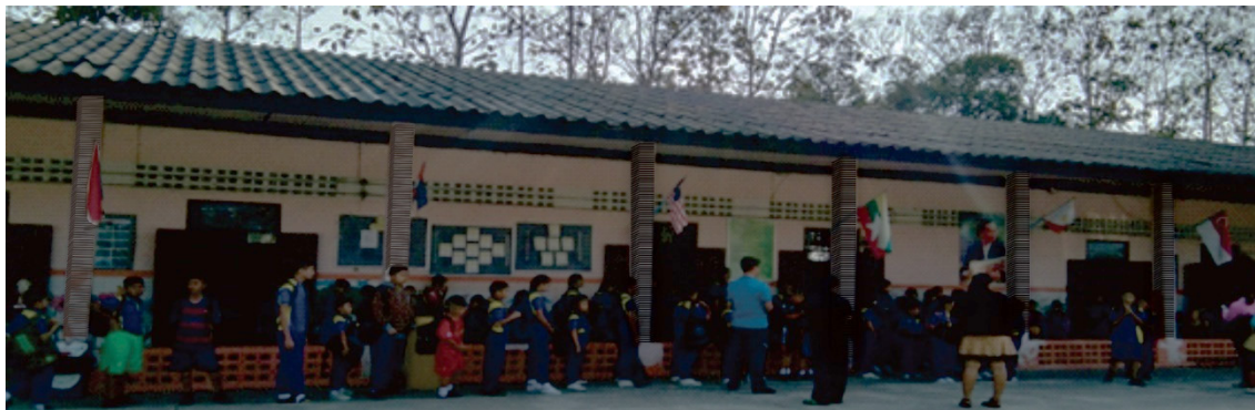
Figure 9 Strengthening of concrete columns after installation of PTMS in the building 1 (front view).
