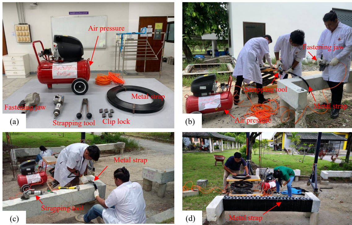
Figure 4 Torsional strengthening procedure: (a) placing a metal strap on the clip lock (b) engaging the strap to the pneumatic strapping tool, (c) applying a tension force to the metal straps along the beam, and (d) beam ready to test.
